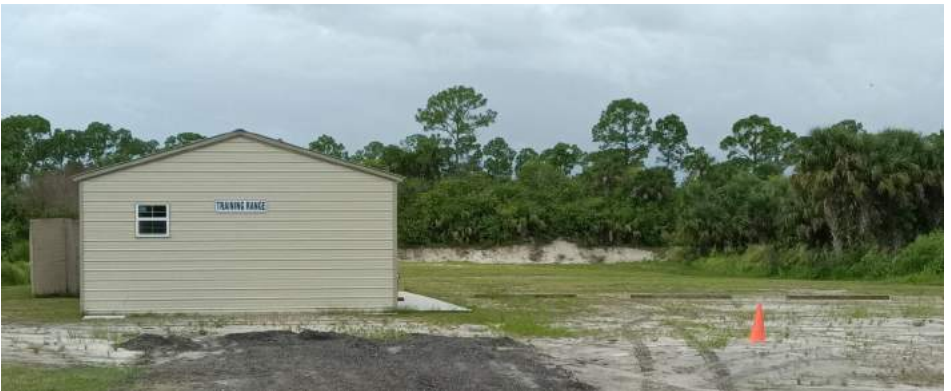
Training Range and Instruction Building
